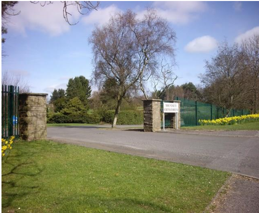
Crematorium front entrance
